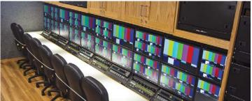
HD-B1 is a 51ft straight unit that was custom designed and built by CSP engineers during the summer of 2014 to fully integrate with HD-4. It provides 12 workstations and is wired for up to three Vizrt CG systems, two 1st-and-10 line systems, two score bugs, and four EVS replay servers. This cutting-edge B unit includes new Cobalt multiviewers and a Utah Scientific  $144 \times 144$  router which has the ability to pass 98 signals between the A and B units over fiber.
